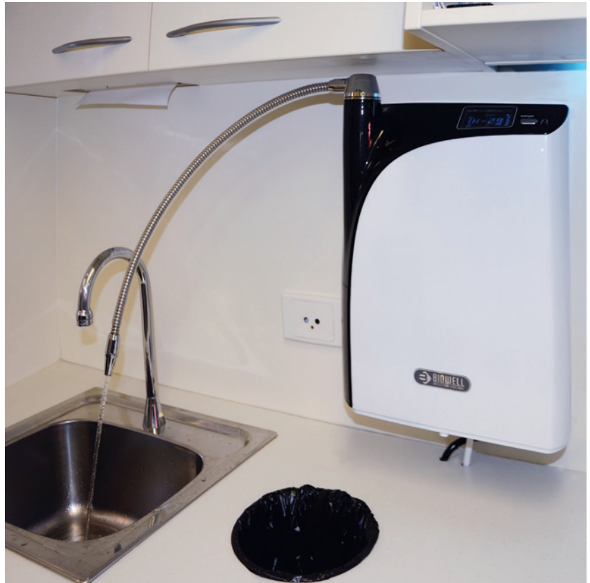
Ozonated water from the Biowell system is used in the dental unit water bottles throughout the day at the practice. It disinfects without leaving a chemical residue or by-product. At the end of the day, a bucket of freshly ozonated water is also sucked through each surgery’s suction lines, before the usual cleaning agent.
